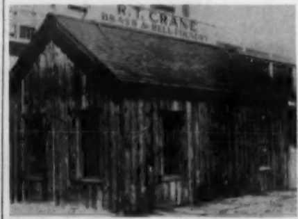
LOG CABIN DAYS—This shack, built by the Crane Co.'s founder, was its first plant. Today it occupies a spot in the midst of the Chicago works.
